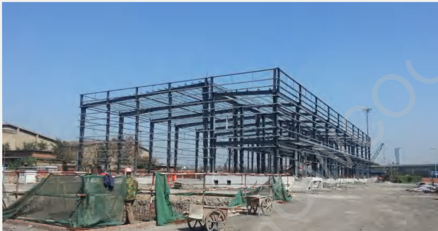
Main structure of large steel cold storage
