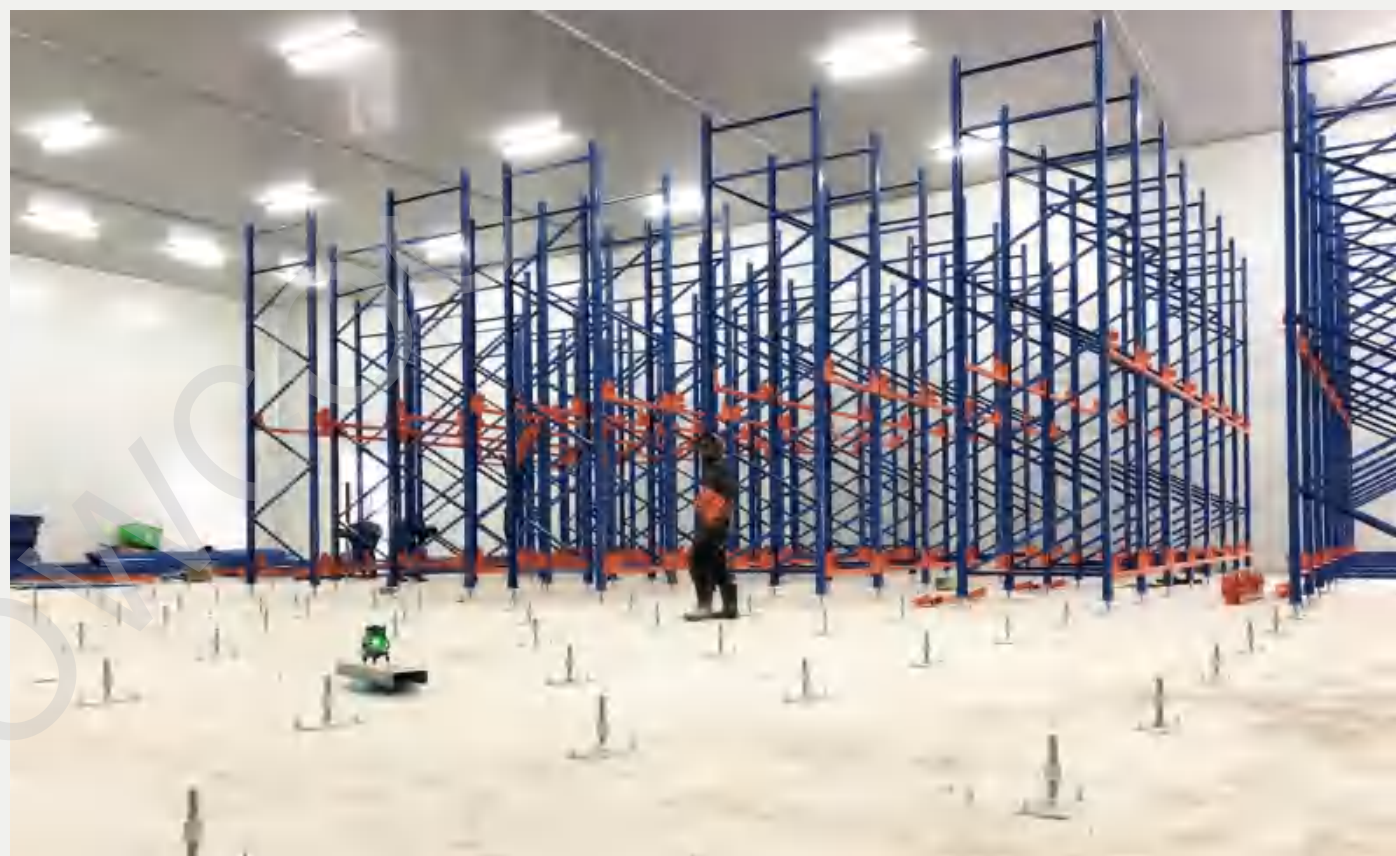
Shuttle Rack Installation
