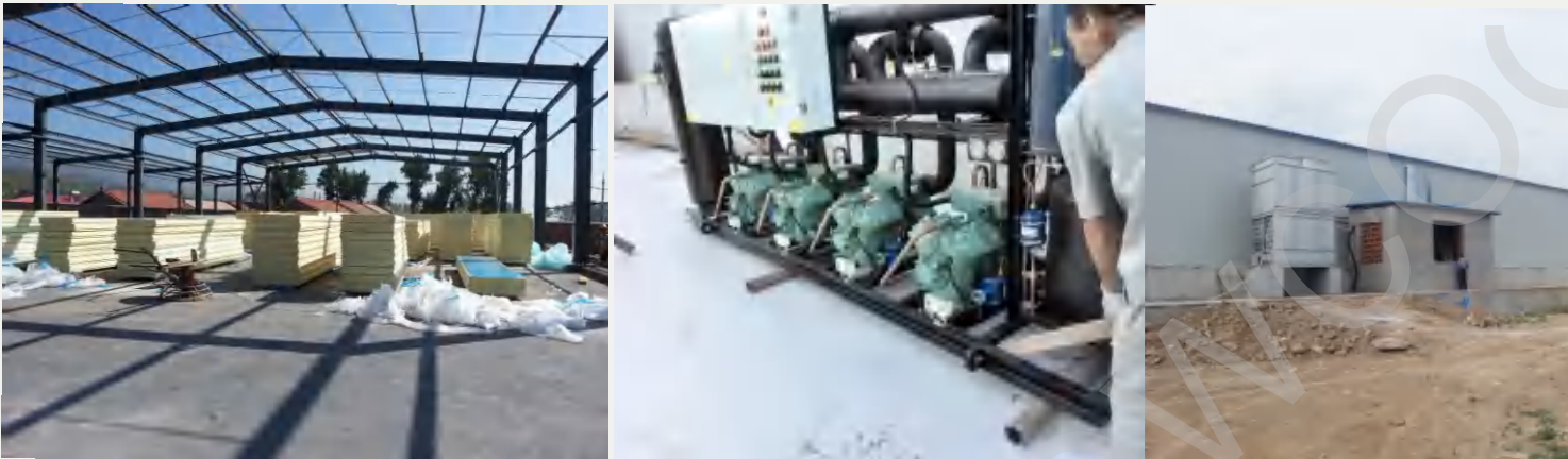
StructureParallel Reciprocating Refrigeration UnitEvaporative Condenser
