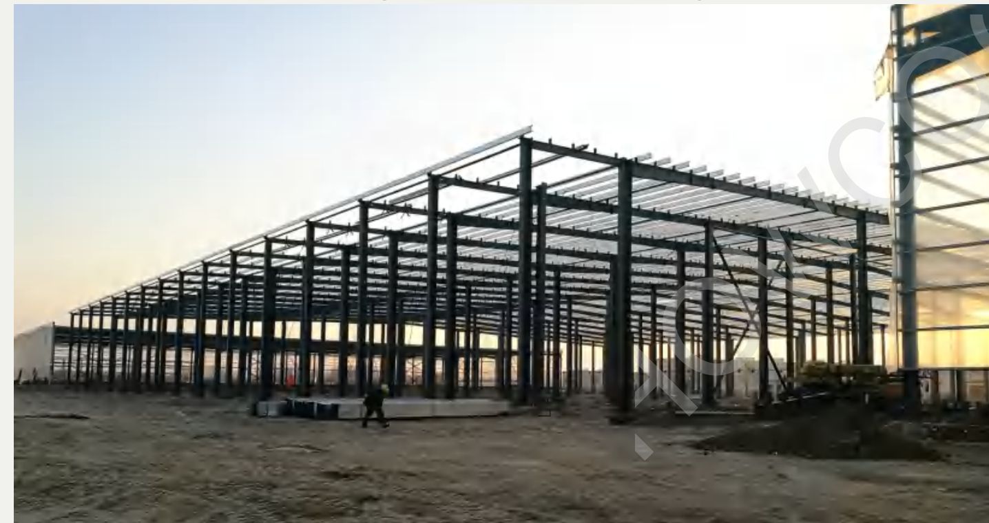
Main structure of large steel cold storage
