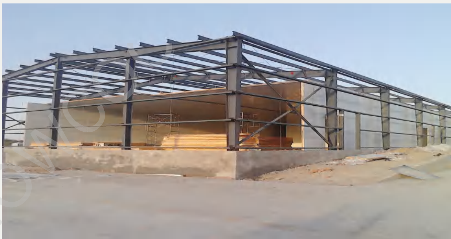
Main structure of large steel cold storage
